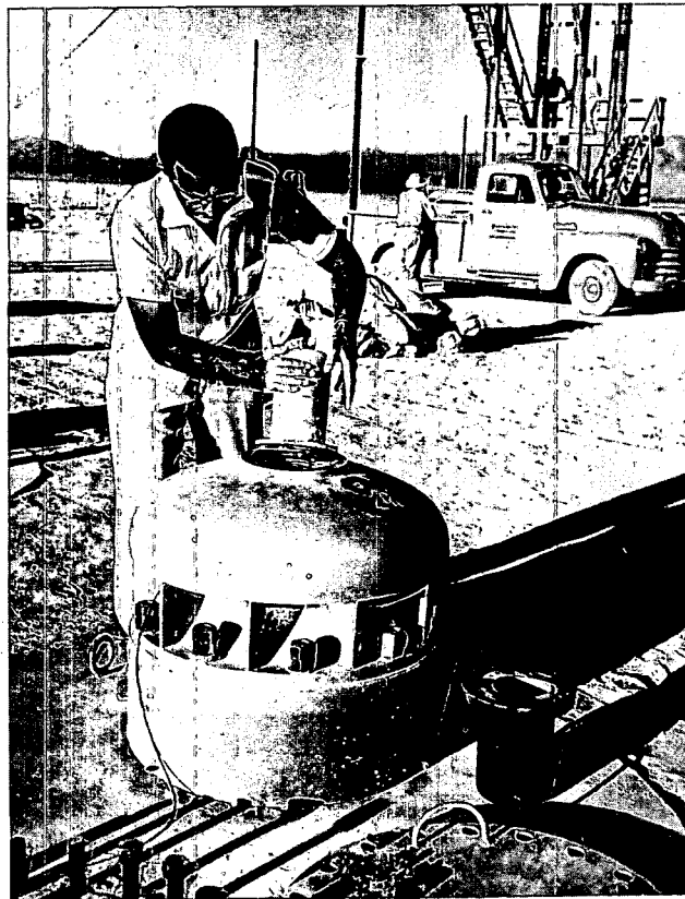
Fig. 4—Placing SR/PT gauge on top of blast valve.
